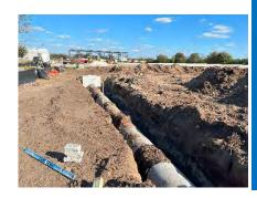
Preferred Drilling Solutions, Inc. (PDS) was contracted by a private developer to install approximately 1,100 linear feet of reinforced concrete stormwater piping at a property contaminated with PCBs. The site was undergoing development into a small industrial park, and the stormwater system was being installed to drain asphalt capped soil impoundments that contained PCB contaminated media.
