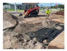
minimum of 98% of modified proctor density, and site restoration with asphalt pavement to match surrounding grade. The work was completed in two days on site.
