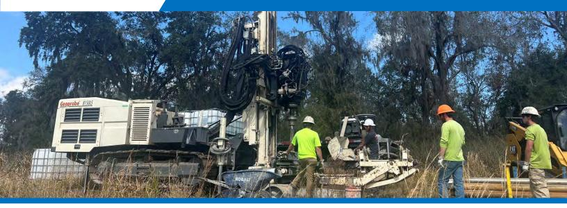
As a member of your project team, Preferred Drilling Solutions, Inc. (PDS) can provide the equipment and services to rapidly assess subsurface conditions in any type of lithology. By utilizing one of our seven (7) state-of-the-art sonic drilling rigs, we can rapidly collect high quality samples, reach deeper depths than conventional auger techniques, and generate less waste.
